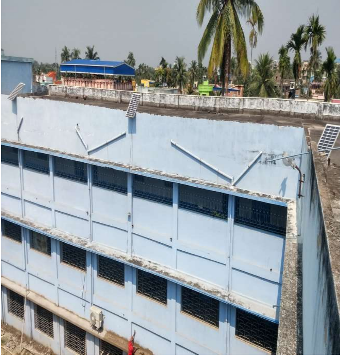
Solar Panels planted on the roof of the college
